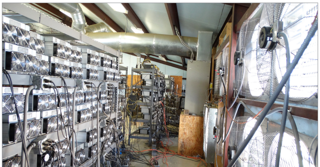
First location mining hardware on the metal shelving and exhaust fans on the right. Picture credit Envista Forensics.
