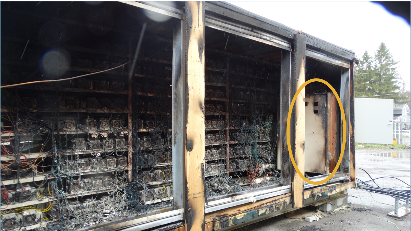
The power distribution panel in the affected container. Picture credit Envista Forensics.
